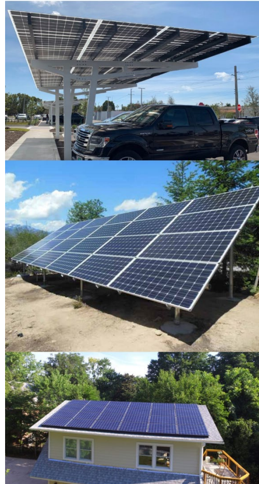
Figures 2 – 4: Top: Building Integrated System (Source: imobipro.com) Middle: Ground Mounted System (Source: unboundsolar.com) Bottom: Roof Mounted System (Source: southern-energy.com)
